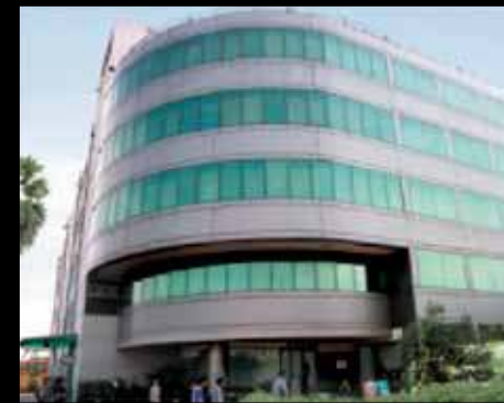
2003 BAANI - IBM, GURGAON
